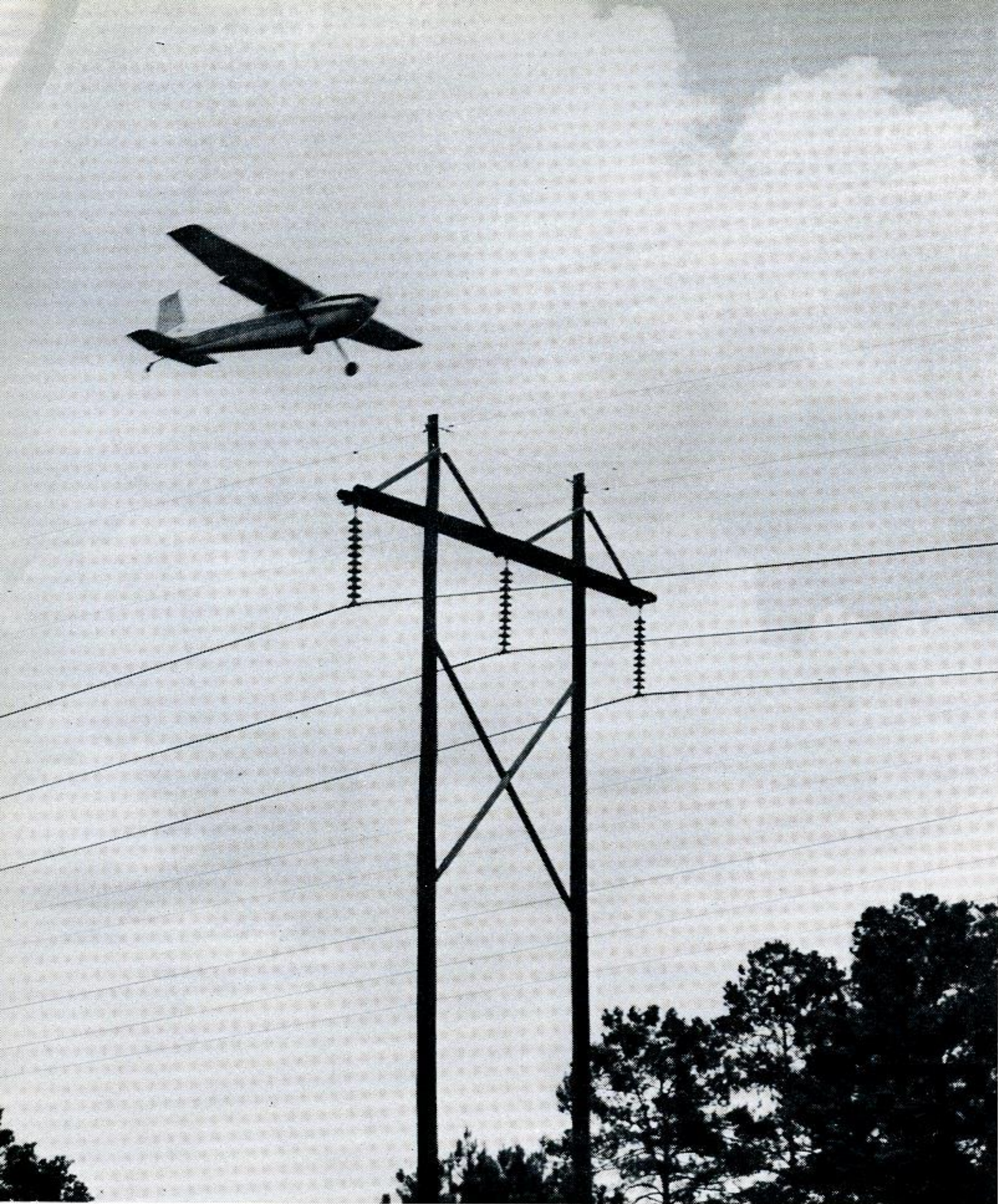
ON TOP OF THE SITUATION. Our Company's "sky patrol" rides the wires close while checking for trouble spots along our numerous miles of right-of-way in the 45 counties and parishes Gulf States serves in Texas and Louisiana.
