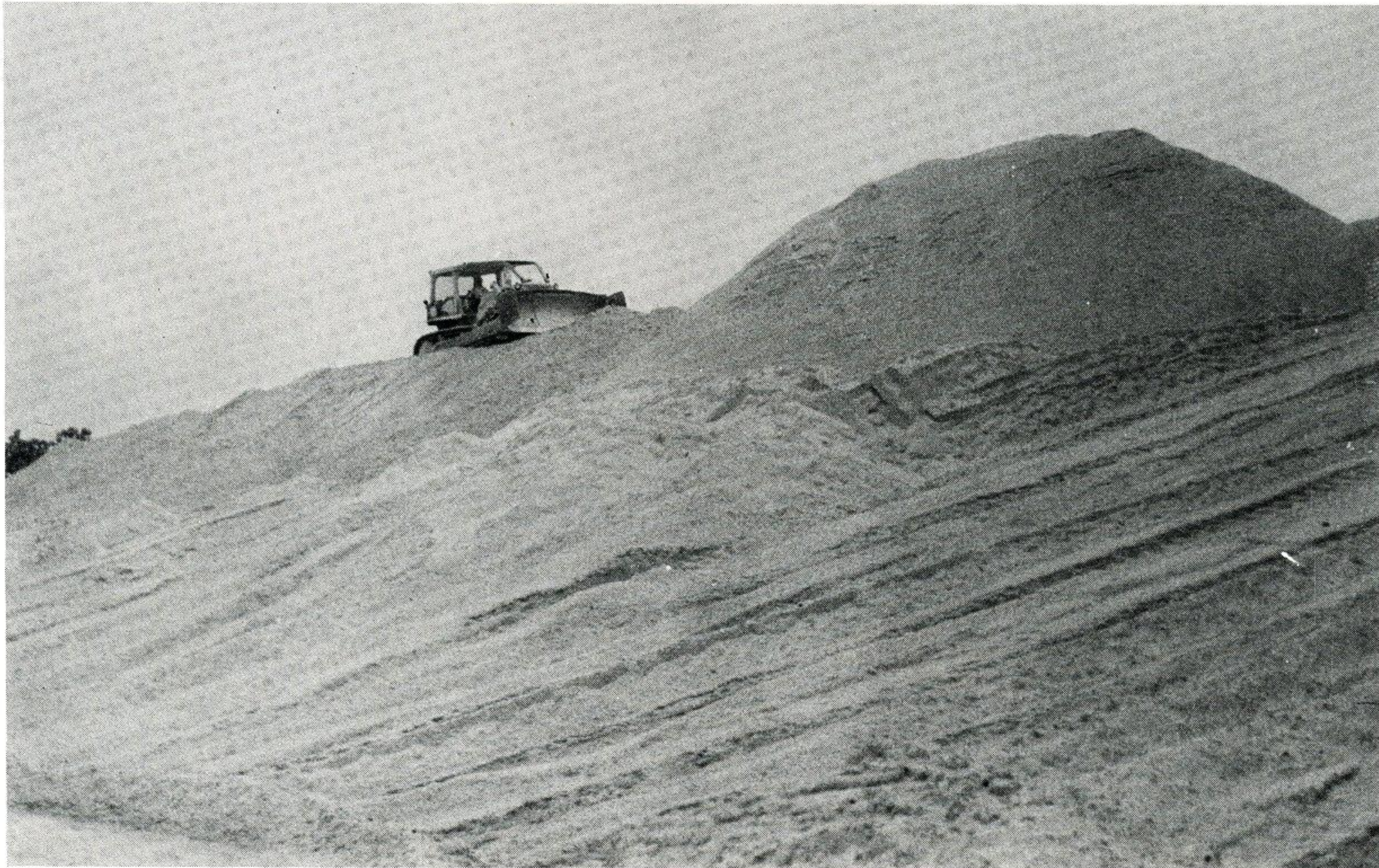
A large portion of the 2.2 million cubic yards of engineered backfill material needed to be placed in the excavation prior to construction is already on hand at the River Bend site. The material must be placed in the hole one layer at a time, compacted, then recovered with another layer.
