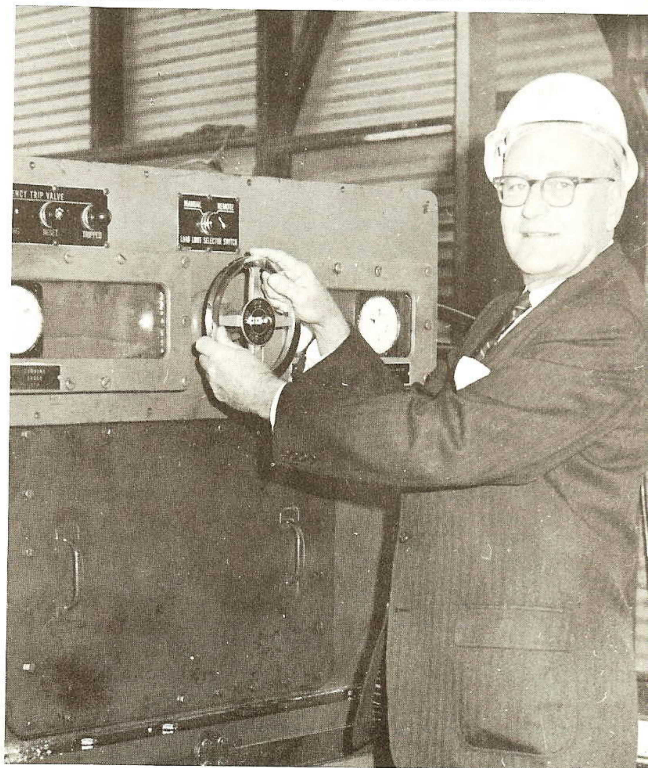
PUTTING 200,000 KILOWATTS ON THE LINE. E. A. Werner, vice president and manager of Baton Rouge Division, adjusts the throttle on a 220,000 kilowatt generator as it is "put on-the-line" at Willow Glen. The estimated $17 million unit took almost two years or approximately 650,000 manhours to install.
