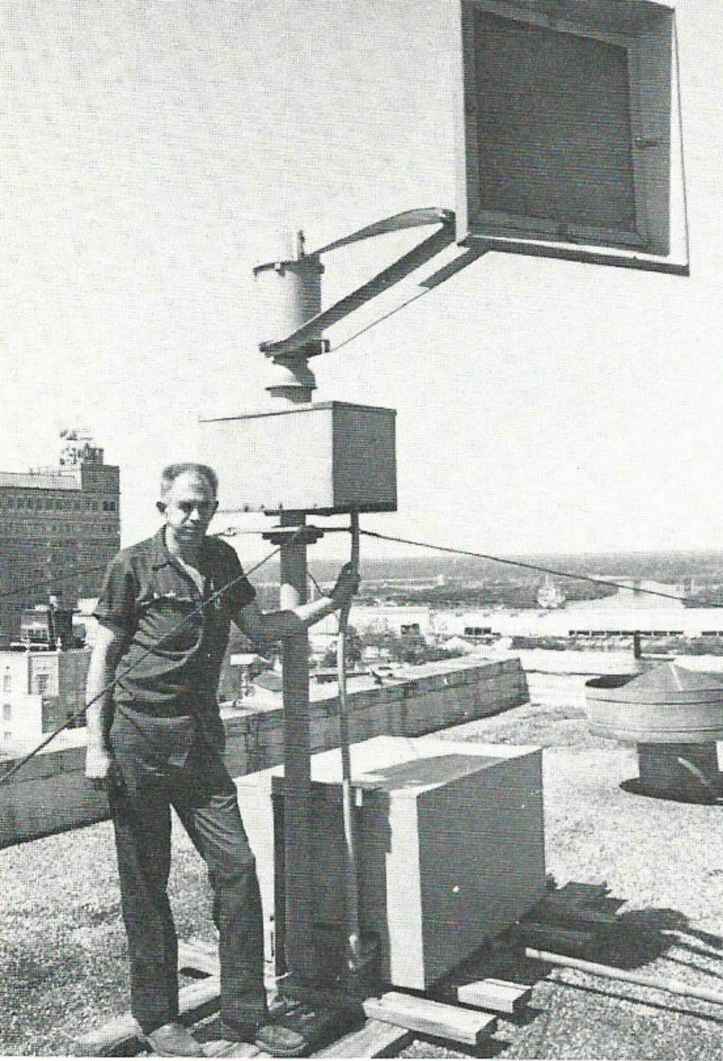
Electrician Ronnie Branch atop the Beaumont Savings Building.
