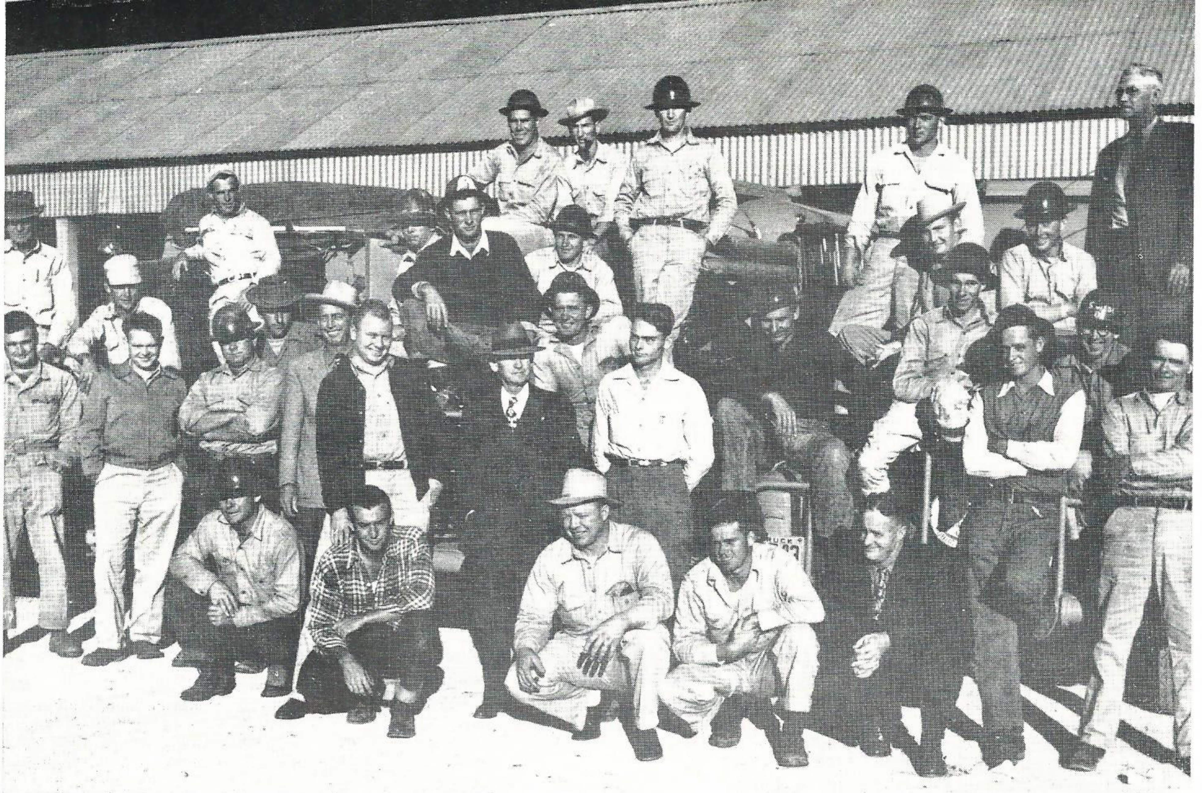
ORANGE T&D—1949. This group picture was made of the employees in the Orange T&D in 1949. Left to right they are: Kneeling, Truman Hodges, lineman; Claude Wilkinson, helper; J. S. Rougeau, serviceman, now service foreman in Orange; Gerald Bridges, lineman, deceased; and C. R. Nantz, now distribution supervisor, Orange; Standing front row: Bil Perry, helper; Dave Lester, engineer; G. W. Dailey, truck driver, Orange; A. L. Stahl, engineer, now right-of-way, Beaumont; Dalton Woodard, appliance repairman, Orange; C. H. "Chief" Meeks, district superintendent, now retired; G. W. Thomas, engineer; Frank Osburn, lineman, Orange; Charlie Brown, truck driver, water
