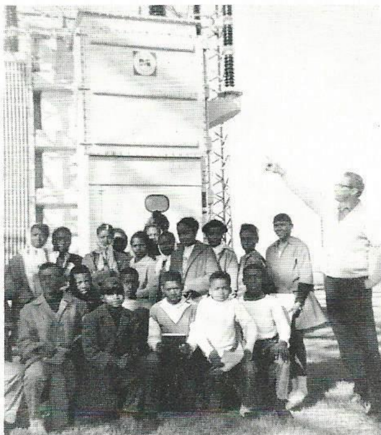
TOUR JENNINGS PROPERTY. Earl Mayfield, substation operator, Jennings, conducts a tour of the Jennings substation for this group of students from the Jeff Davis Training School in Jennings.
