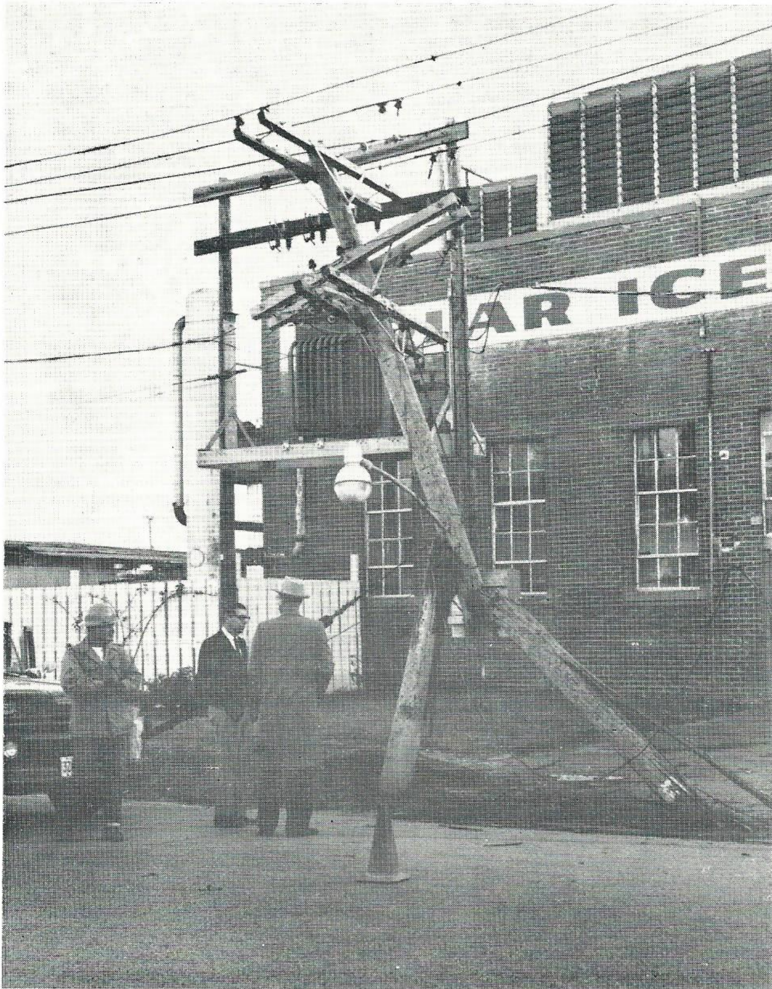
WHAT HAPPENED HERE? Bill Heaner, Claims Department, center, and Floyd Smith, operating superintendent, right, discuss smashed distribution pole just north of the intersection of Pearl and Long in Beaumont one cold morning recently. Looking on is J. E. Lamar, helper T&D. A truck traveling down Pearl, a one-way street into downtown Beaumont, clipped the pole high on the left side, tearing out the middle section which appears as the right-hand leg of an upside-down Y. The butt of the pole, left leg of the Y, is still in the ground while the top is partially held up by lines.
