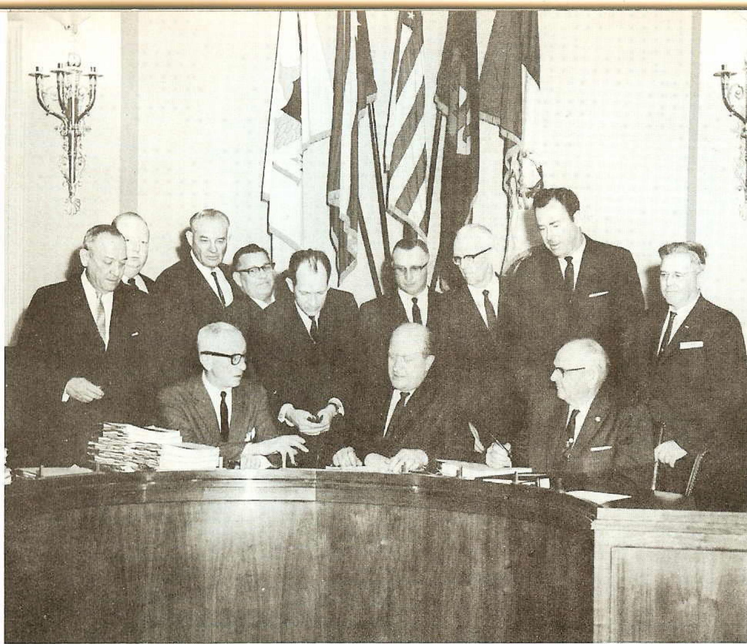
SIGN CONTRACTS FOR SAM RAYBURN DAM ELECTRIC POWER. W. H. Gieseke, standing far left, vice president and secretary of our Company, and Chairman Morrison, seated left, were among the signers of the contracts signed last month in Washington for electric power to be generated at the new Sam Rayburn Dam on the Angelina River. The nine 20-year contracts signed will enable power to be sold from the Southwestern Power Administration via the Sam Rayburn Dam Electric Cooperative. In turn, these agencies will sell power to our Company which will, in turn, furnish it to local systems. Present for the signing were: Mr. Morrison; Kenneth Holum, assistant secretary of interior for water and power development; Clyde Wainwright, president of the board of Sam Houston Electric Cooperative; Mr. Gieseke; Robert Willis, mayor of Livingston, Texas; Douglas Wright, administrator of the Southwestern Power Administration; W. A. Venissat, mayor of Vinton, Louisiana; Congressman Jack Brooks of Beaumont; J. W. Withers, president of the board of the Jasper-Newton Electric Cooperative in Kirbyville; M. P. Hancock, mayor of Jasper; Dempsey Henley, mayor of Liberty; and Louis Stanford, secretary of the board of the Sam Houston Cooperative.
