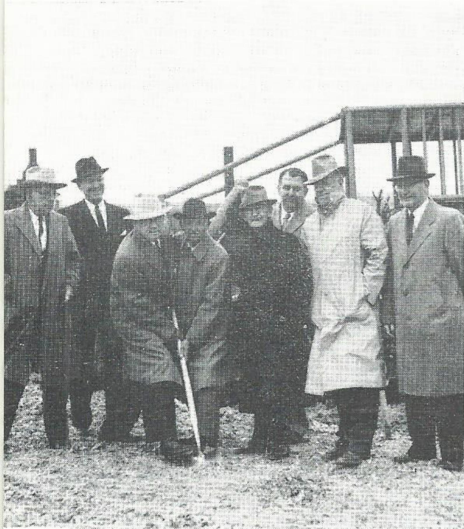
FROM THIS . . . Mr. Nelson turns first shovel of dirt at Sabine site as Orange County leaders look on. Groundbreaking took place on March 17, 1960.
