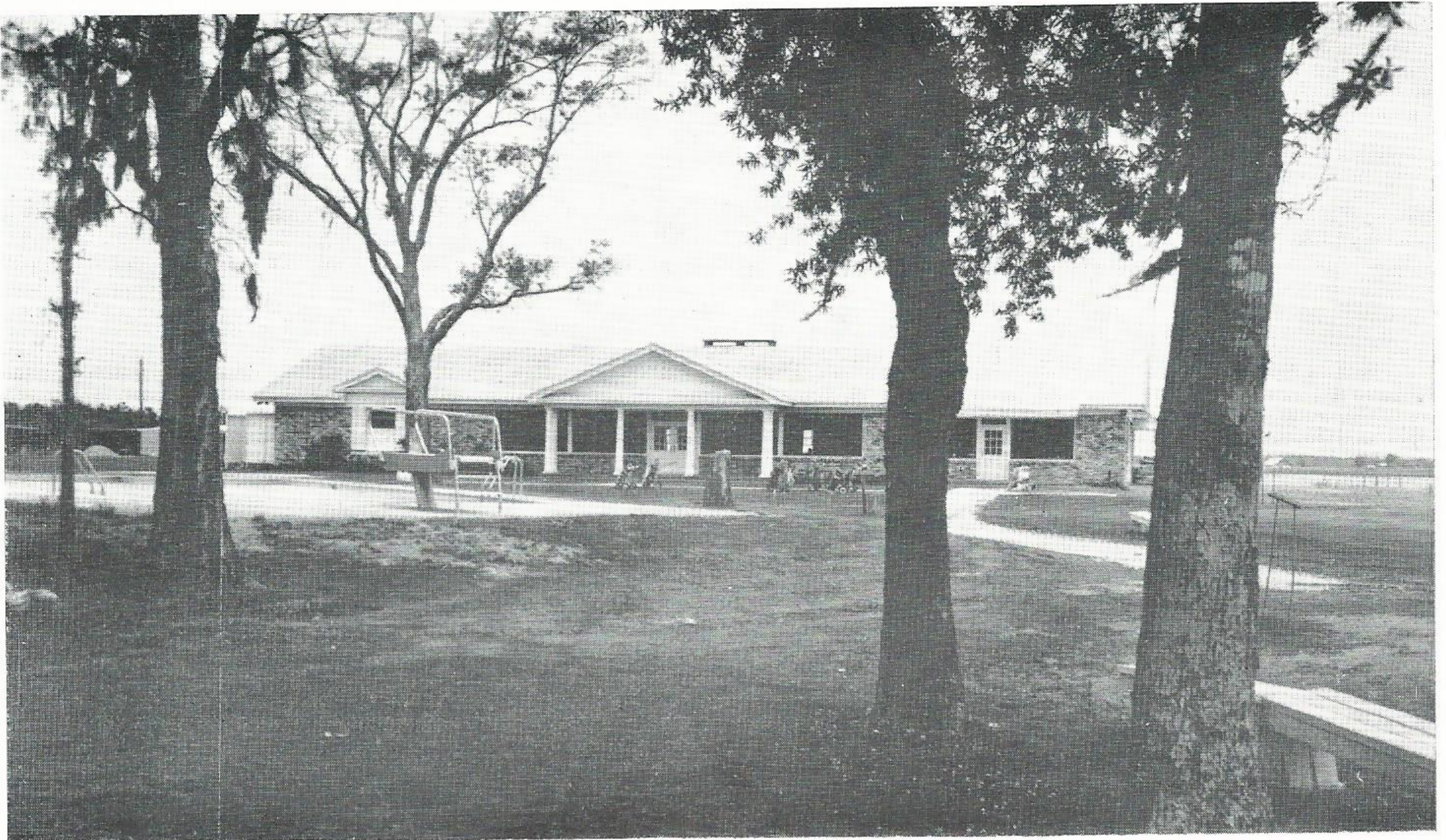
SITE OF 1962 EMPLOYEES' GOLF TOURNAMENT. On Memorial Day, May 30, the club house, swimming pool and entire facilities of the Bayou Din Golf Club on LaBelle Road in Beaumont will be available
