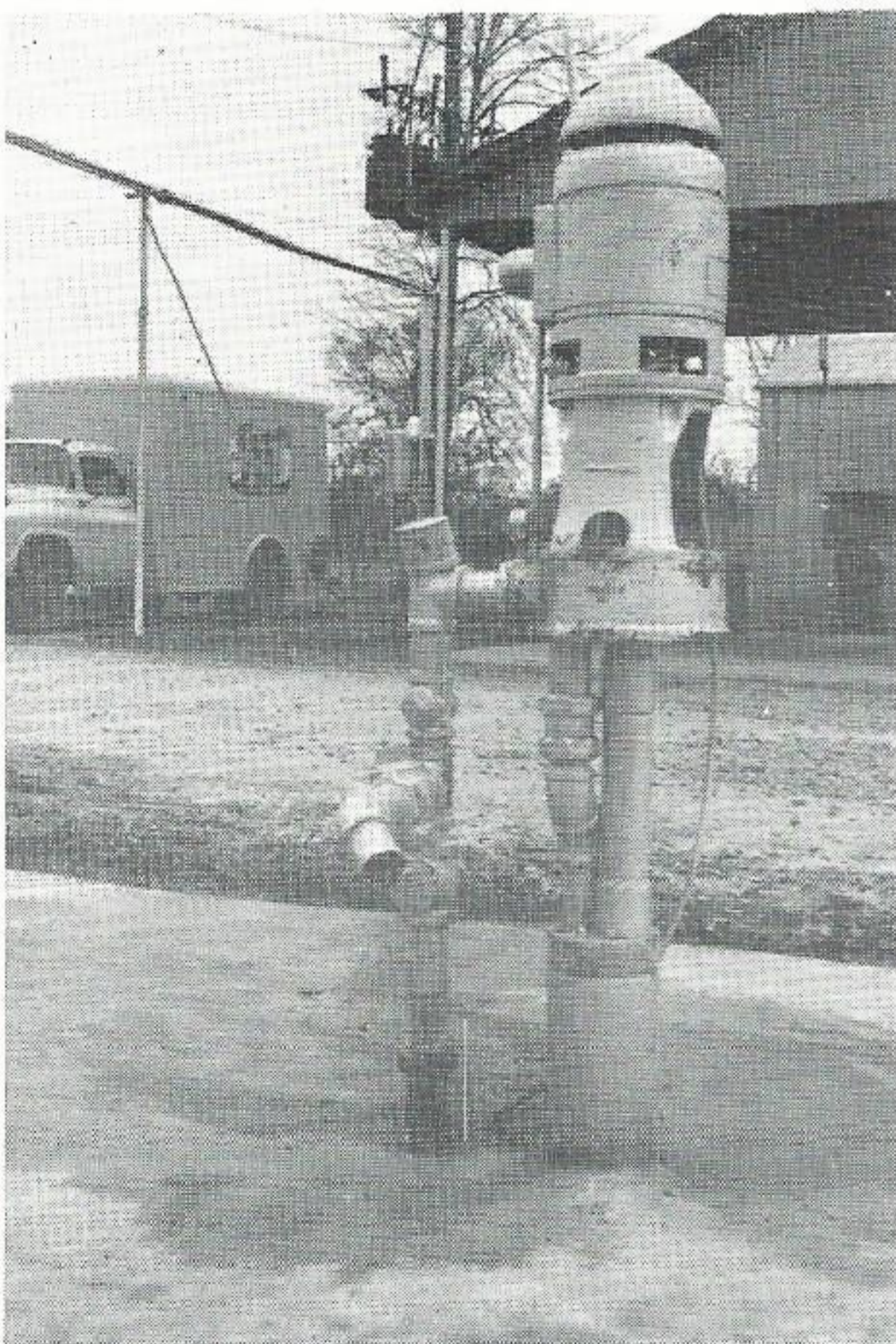
PLENTIFUL WATER SUPPLY. Powered by a five horsepower, three phase electric motor, this pump can deliver 1,500 gallons of water an hour from the 400 feet well at Kleinpeter Farms Dairy.
