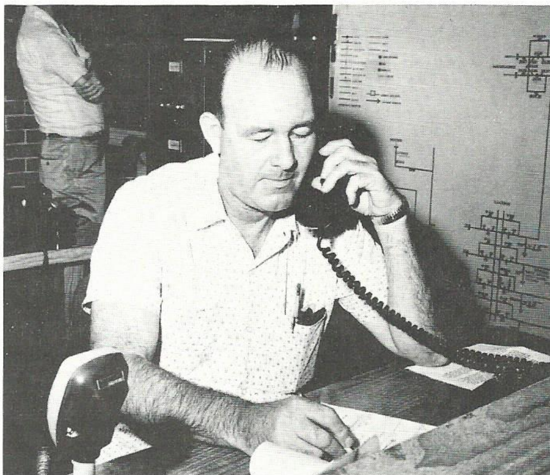
LISTEN ATTENTIVELY. J. L. Poole, Port Arthur T&D, pays close attention to a call to be sure he gets all necessary information correct before he makes any changes on the Port Arthur dispatching board.
