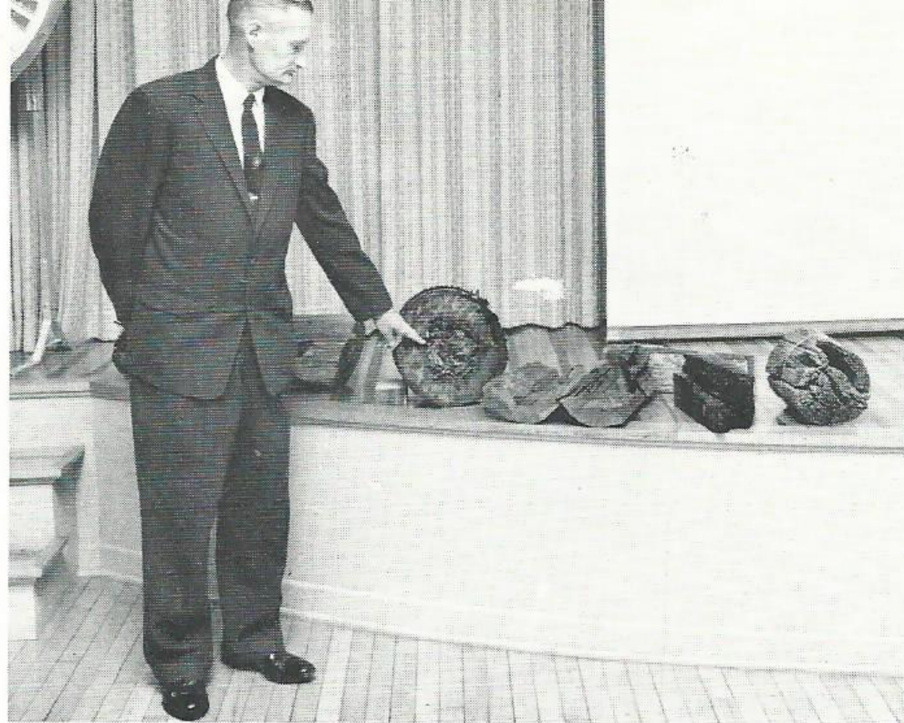
POLE DAMAGE CAUSED BY ROT. A. W. Baird, operating superintendent, Navasota Division, points out the rot damage in these cross sections of poles at the October department head meetings.
