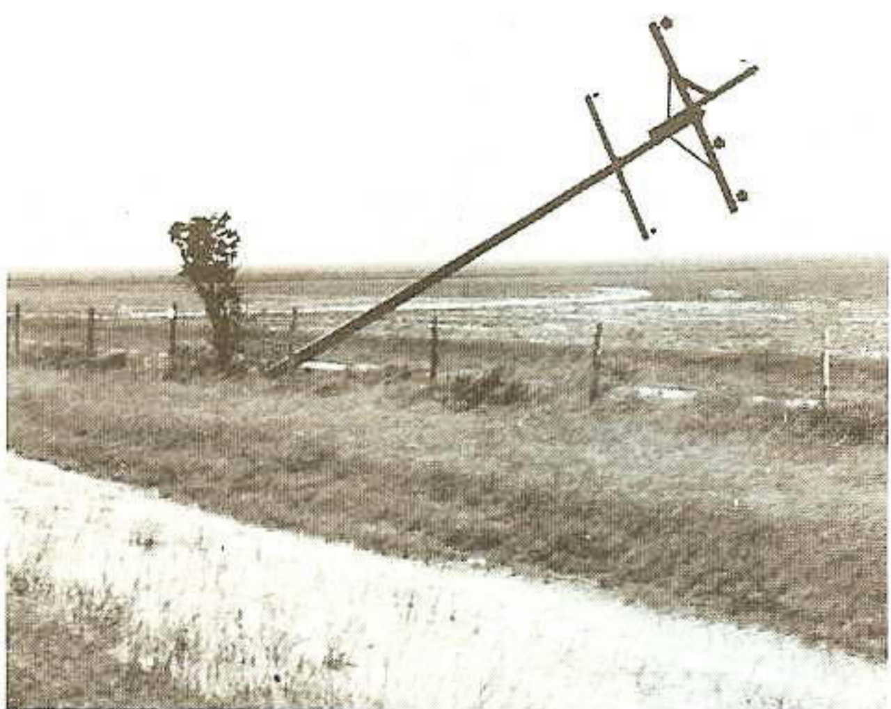
ANOTHER ONE GOES DOWN. Another of our Company's transmission poles bows to Cindy's forces just east of Anahuac. Scenes like this were repeated several times as the storm moved inland Tuesday, September 17.
