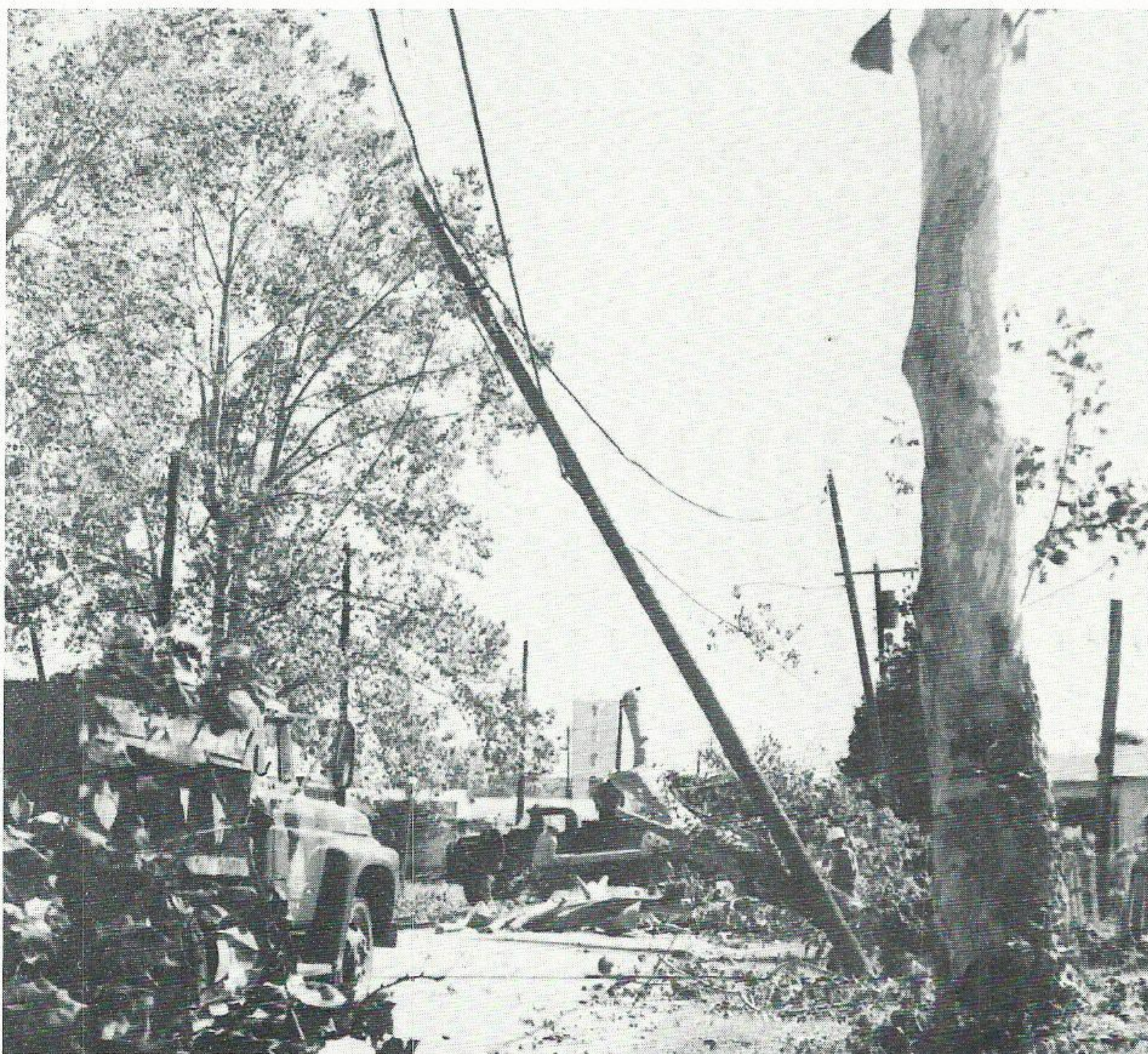
... wind and trees caused extensive damage in Baton Rouge Division.
