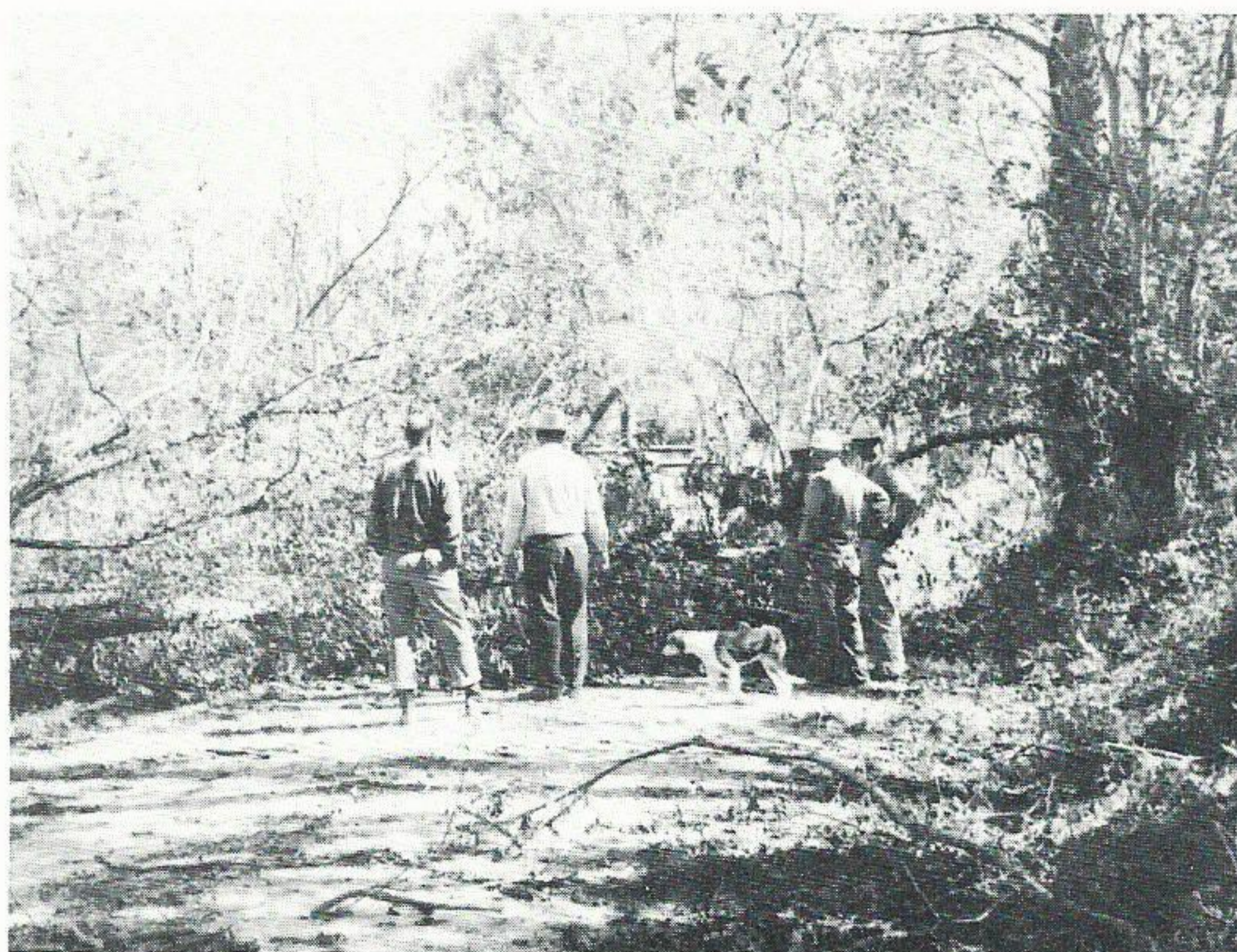
. . . crews attack trees in Baton Rouge area.
