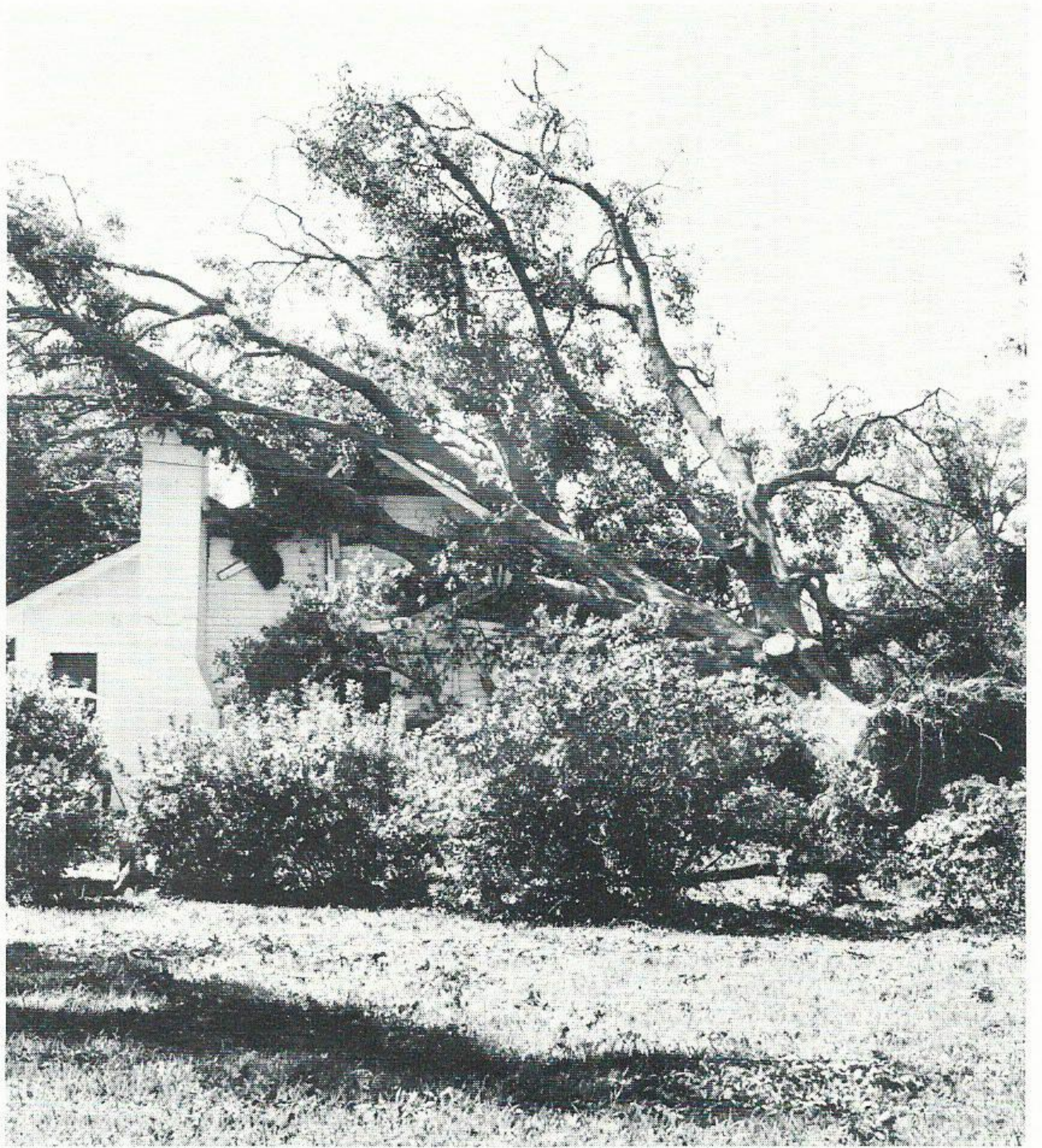
. . . falling trees heavily damage Lafayette District home.
