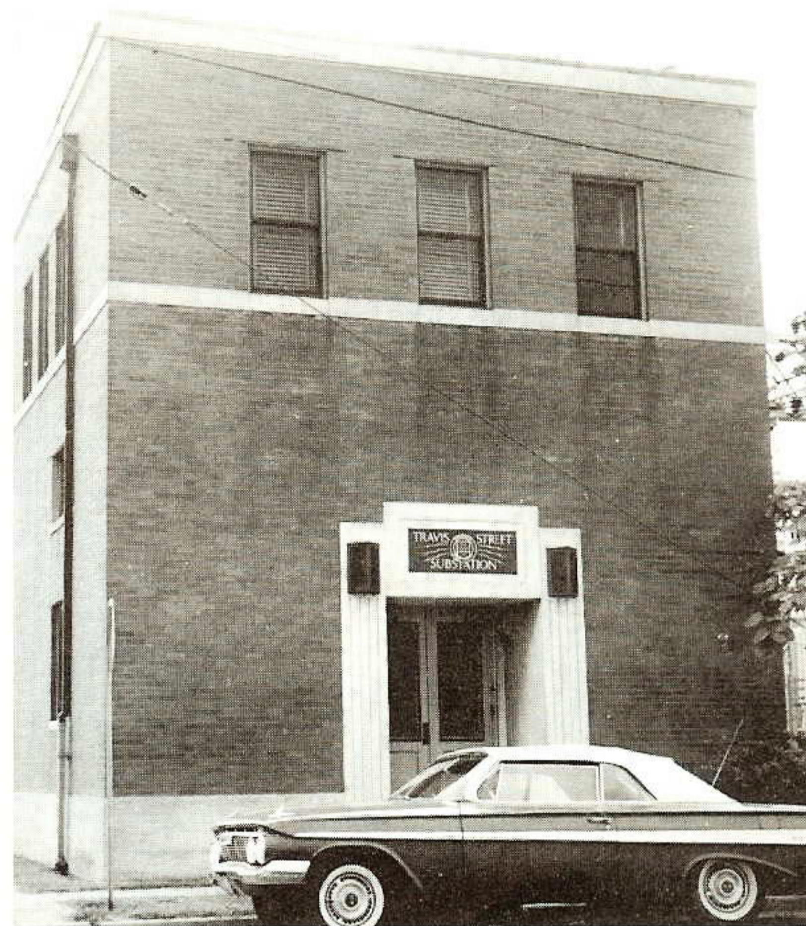
HOUSED SYSTEM DISPATCHERS. This brick building at the Travis Street Substation housed the system operators on its second floor for more than four decades.
