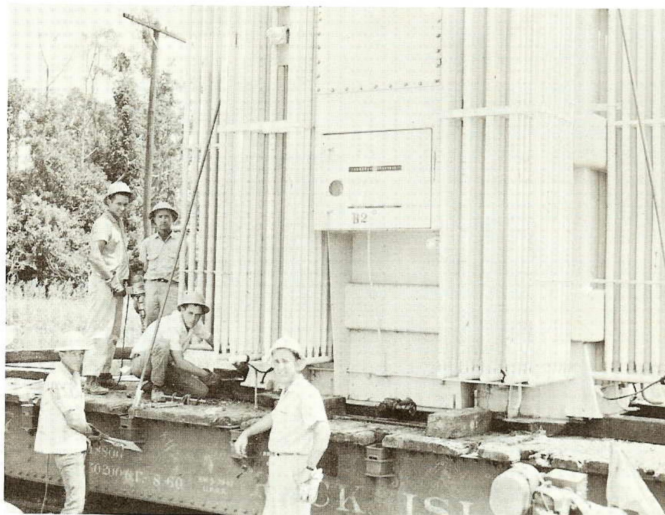
TRANSFORMER ON THE MOVE. A Lafayette substation crew prepares a 7,500 KVA transformer at Sunset, Louisiana, for shipment to Beaumont. The transformer had been taken out of service at the Sunset substation. Members of the crew are, Bill McFarlin, Rayford Bertrand, Wilfred Duhon, George Arceneaux and Charlie Breaux.
