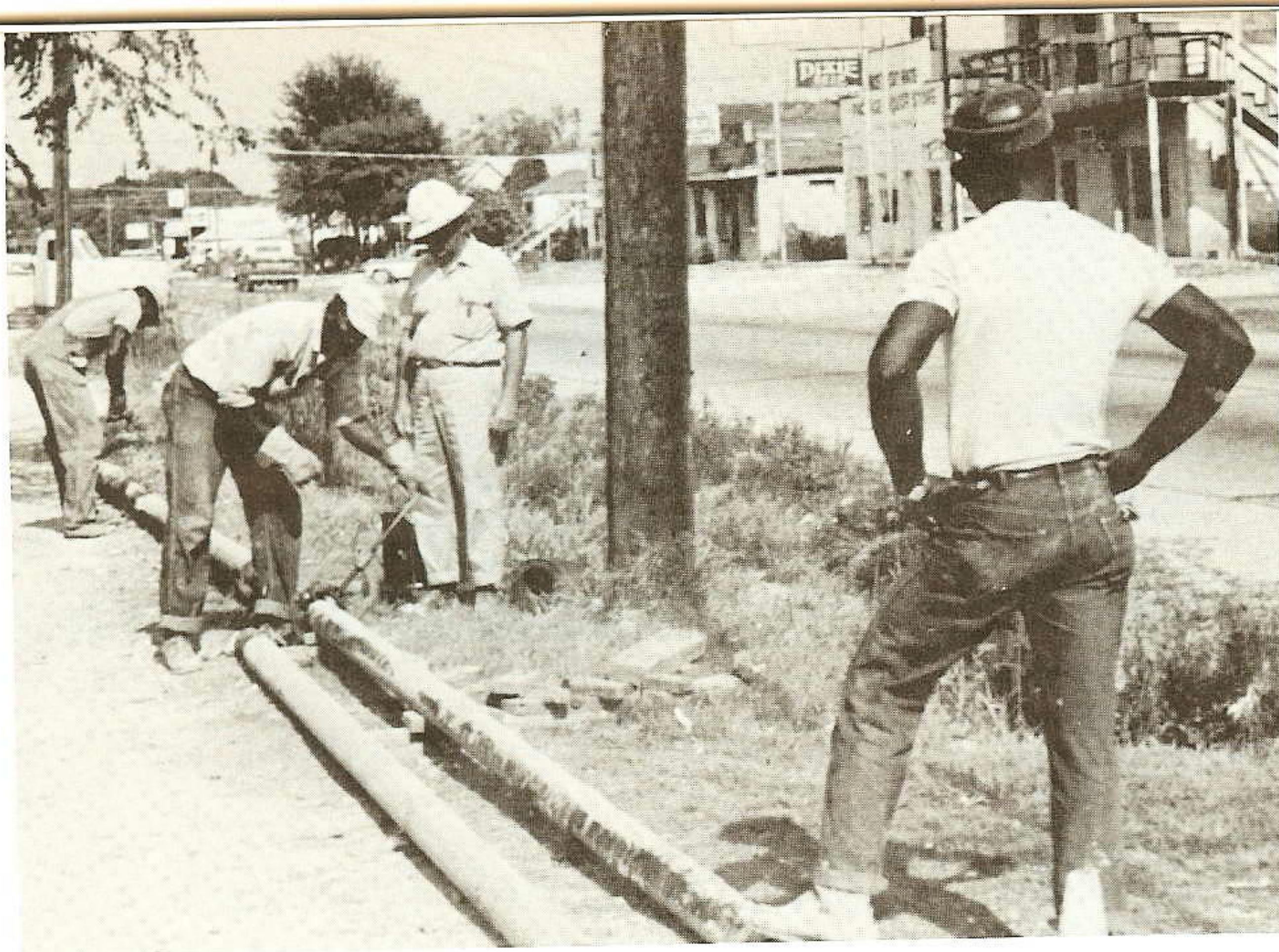
REPAIRS MAIN. The crew of J. A. Leteff, gas foreman, center, cut up a section of gas main that they have replaced. They had to replace some 70 feet of pipe that had been attacked by electrolysis. Members of the crew shown are, left, Booker T. Washington, Sevear Young and Joe Blakes. Replacing mains is one job that must wait for warm weather. If a leak is discovered in the winter, temporary repairs are made to maintain service.
