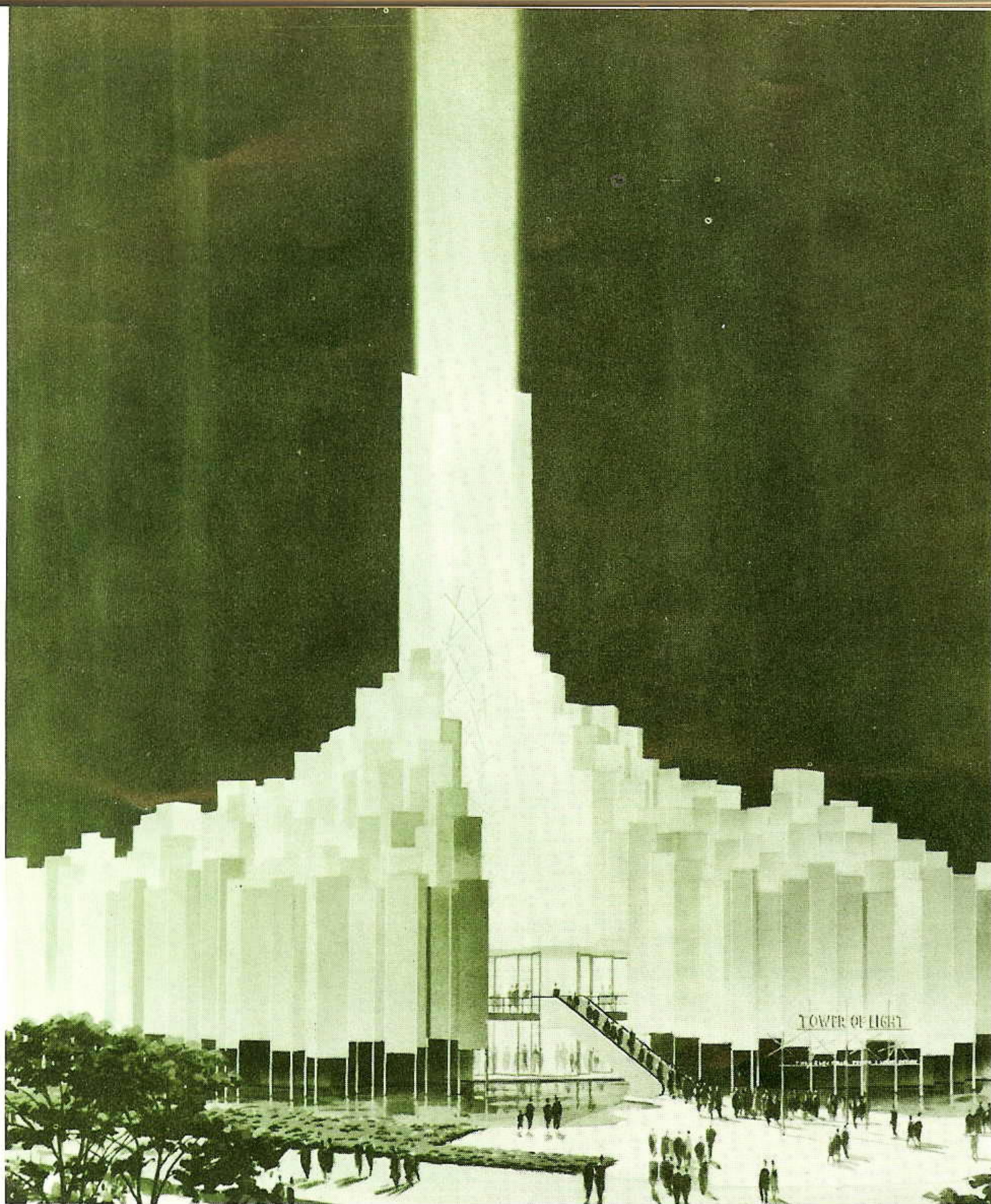
TOWER OF LIGHT. The investor-owned electric utility companies' exhibit will be housed in the Tower of Light Pavilion which has been constructed of vertically staggered anodized aluminum panels rising, like an irregular pyramid, to a peak of 80 feet. The center of the building is an open light court from which three 120-foot high prismatic pylons extend to frame a shaft of light beamed skyward. Inside, visitors will be treated to a gay musical show that tells the story of the investor-owned electric utility industry and free enterprise.
