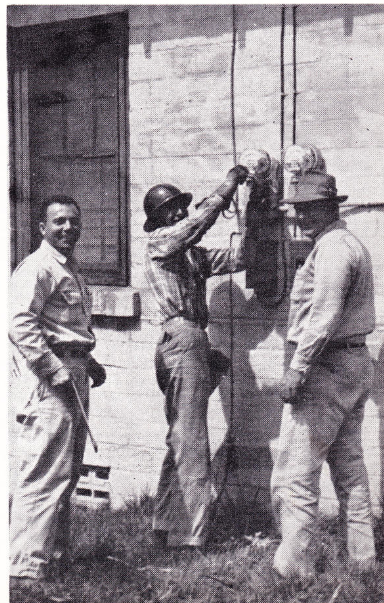
METERS are installed on a duplex at Weeks by Paul Dugas, John Beaugh and Kelley Powell preparatory to switching customers over to GSU's distribution system.
