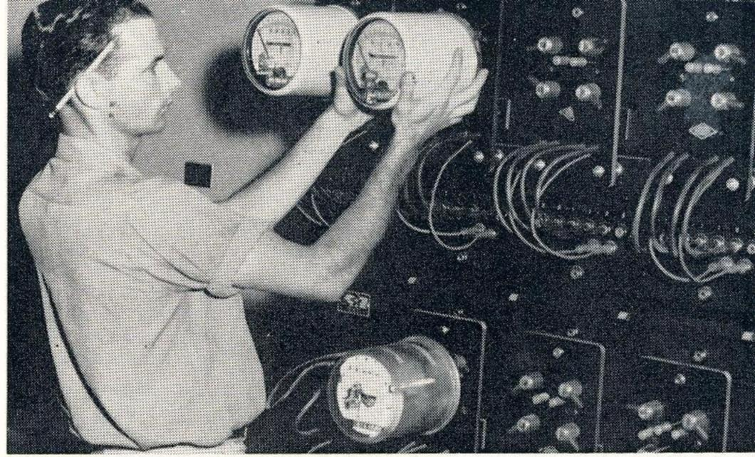
This is a "gang-testing board," which is capable of testing from one to 23 load meters at a time. Meters are run on this board for about 45 minutes under full load to determine their accuracy. The meter at bottom is a master, with which the others must conform.
