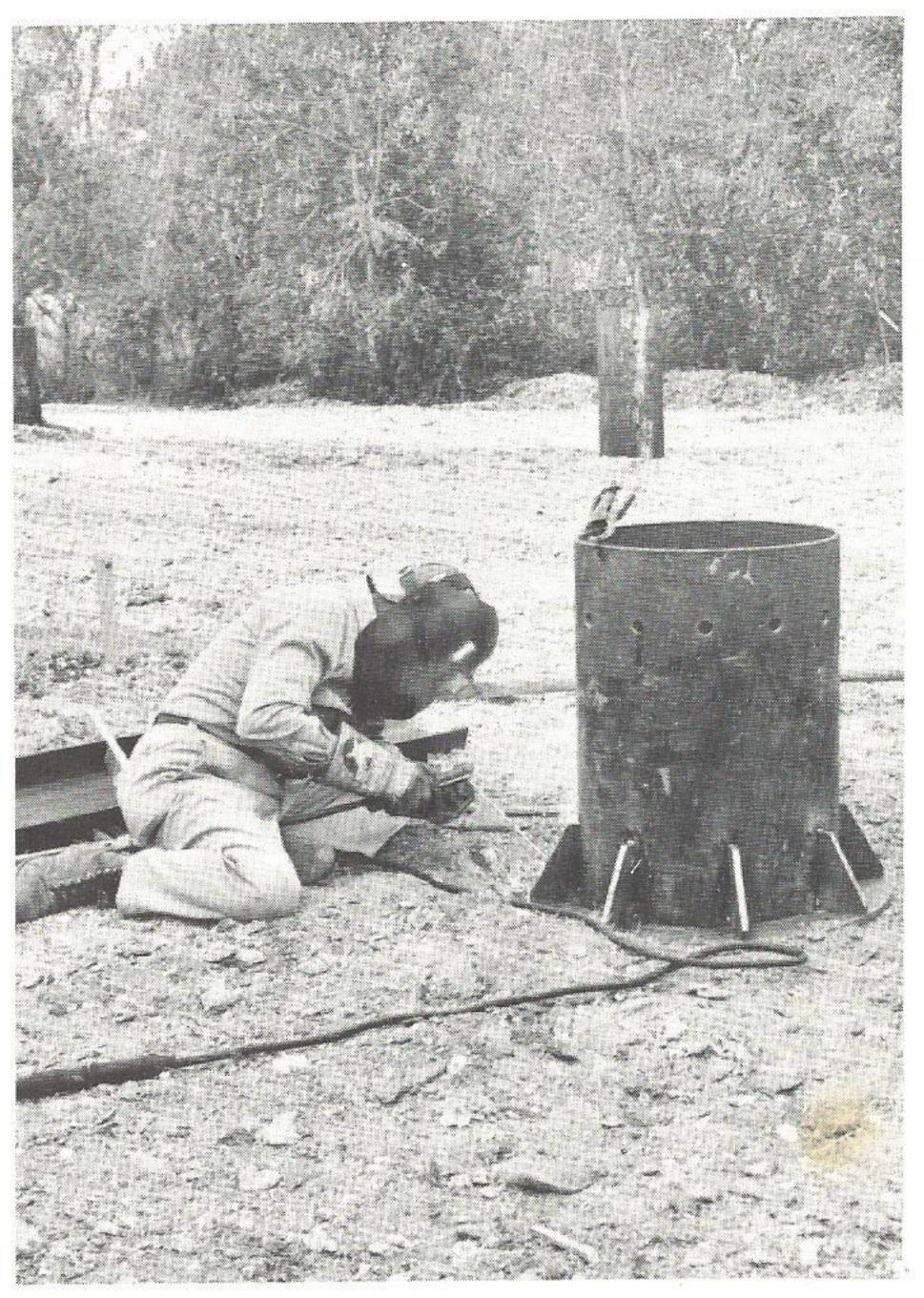
Supporting brace for experimental pole is welded on here, but a bolt-on brace has been developed for future use. This is part of the tests conducted at Lindbergh.
