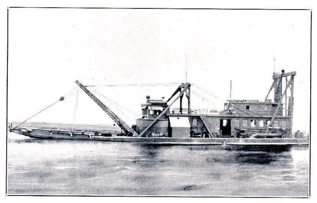
This is the Standard Dredging Company's hydraulic dredge Windham, which will soon begin nosing its way through the salt marshes in the south end of Jefferson County, leaving in its wake a path of water which will be a link in the Intracoastal Canal. Our electricity will turn the powerful motors that run the pumps that eat out a stretch of marsh some 25 miles long.
