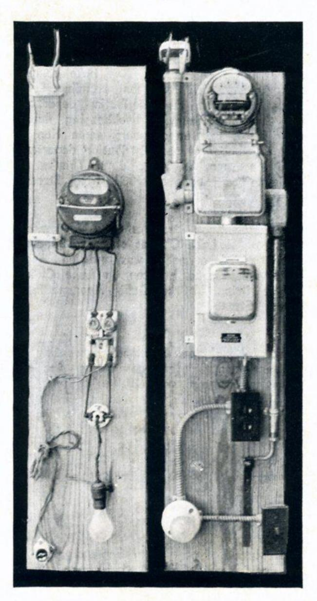
The above meter installations, each mounted on a board, illustrate the old and more or less dangerous open-wiring meter installation, left, as compared to the new method of enclosed wiring job, on the right. These were made up and used by Superintendent Ray Hereford, and other Conroe employees, who were asked to take care of the "electrical side of safety in the
